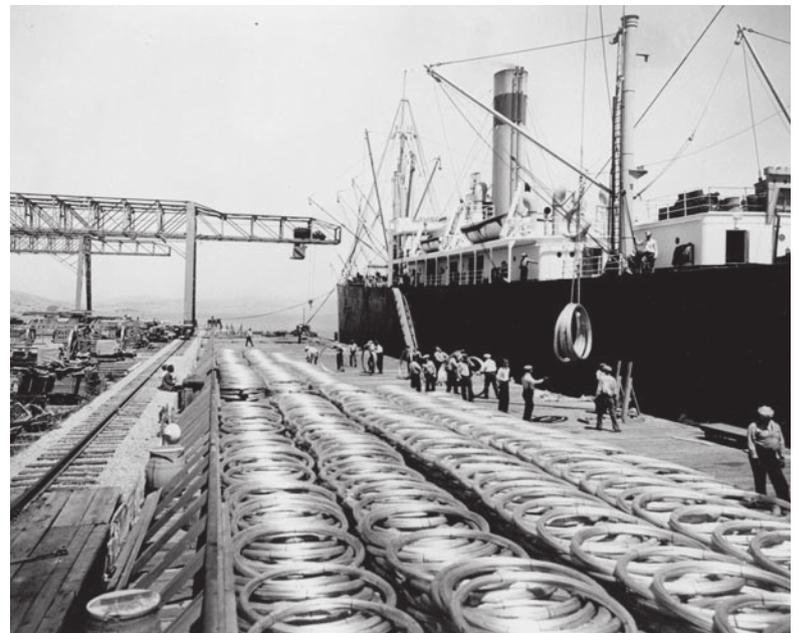
Steel wire from New Jersey was shipped and unloaded on the wharf of the Roebing plant where it was washed, wound and reeled into cables for the Golden Gate Bridge.
