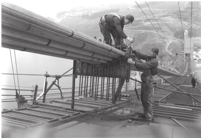
Bridge workers built a catwalk to connect the towers at both sides of the Golden Gate strait so they could attach the suspension cables to hold up the bridge roadway. (Photo: Golden Gate Bridge, Highway & Transportation District)
