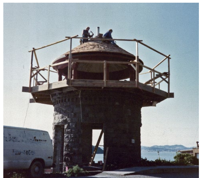
Tower roof restoration in 1984, the last phase of the complete restoration.
