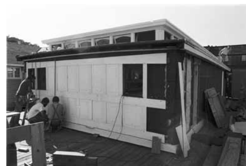
China Cabin’s south wall work March 30, 1981, photo by Phil Molten
