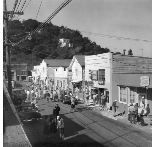
Northwest side of Main in the early stages of the paint-up.
