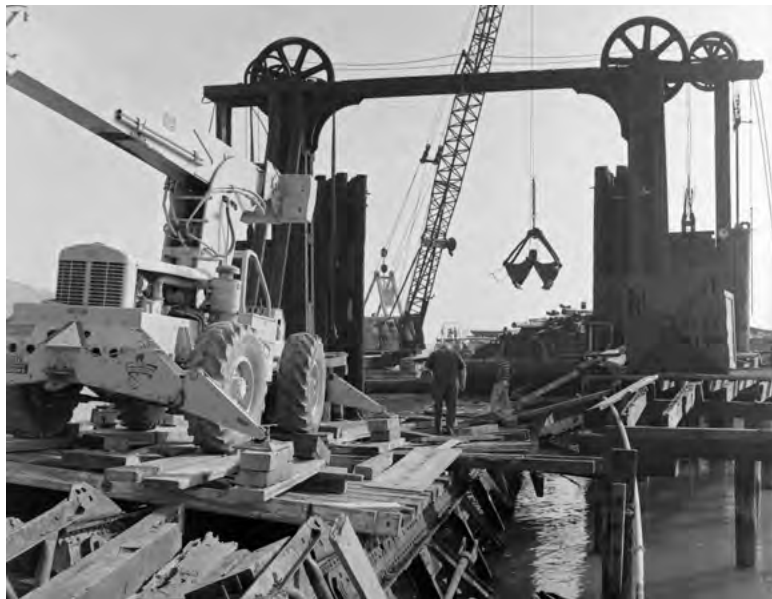
Gallows frame demolition February 1974 (Phil Molton collection)
