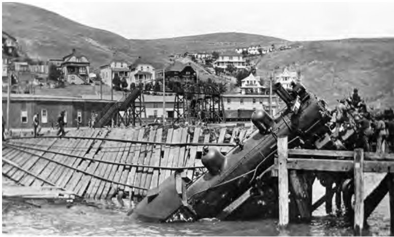
Engine 112 after the dock collapsed in June 1913. Just beyond is the new pedestrian viaduct over the yard to Mar West.
