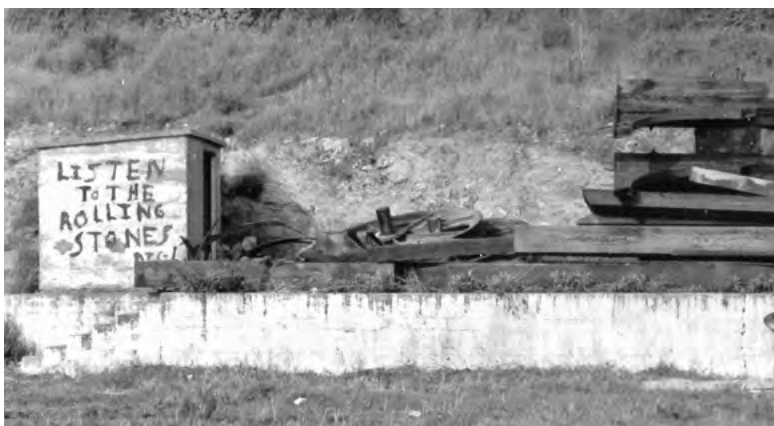
Just below Mar West Street the abandoned railroad yard was good place for artistic photography and graffiti. In the center are the gallows wheels now on display at the Depot Museum.
