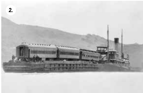
1. Loading three railcars onto a barge at the Tiburon waterfront, 1934.
