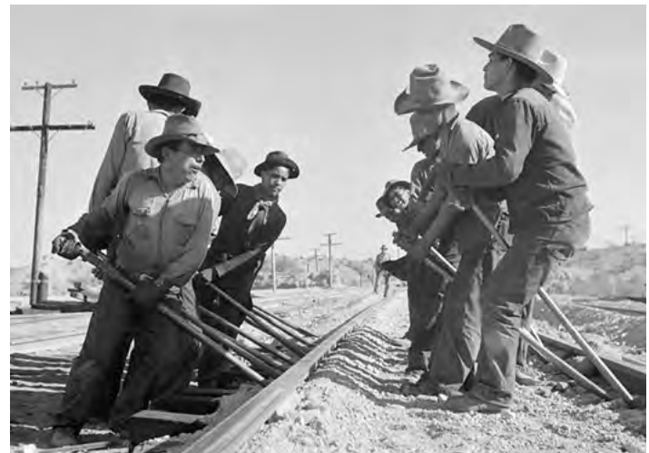
Gandy dancers work in unison using lining bars to align the tracks in 1943. (J. Delano)
