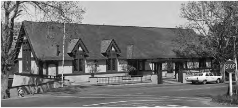
Below: Belvedere City Hall about 20 years after it was rolled down Laurel.
