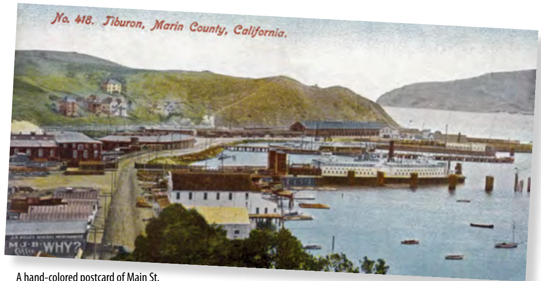
A hand-colored postcard of Main St. and the NWPRR yard circa 1909. On the far side of the yard is the Depot with the long passenger shed next to it. Up front is the Ukiah at the rail car loading dock, which could hold 12 freight cars on the lower deck.
