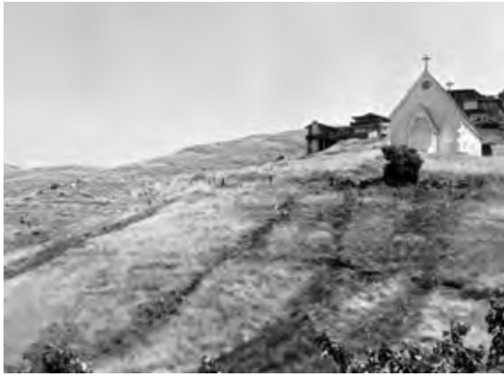
Tiburon's aquifers and underground streams like these shown below Old St. Hilary's provided a source of fresh water for the railroad and growing town but would often dry up in times of drought.
