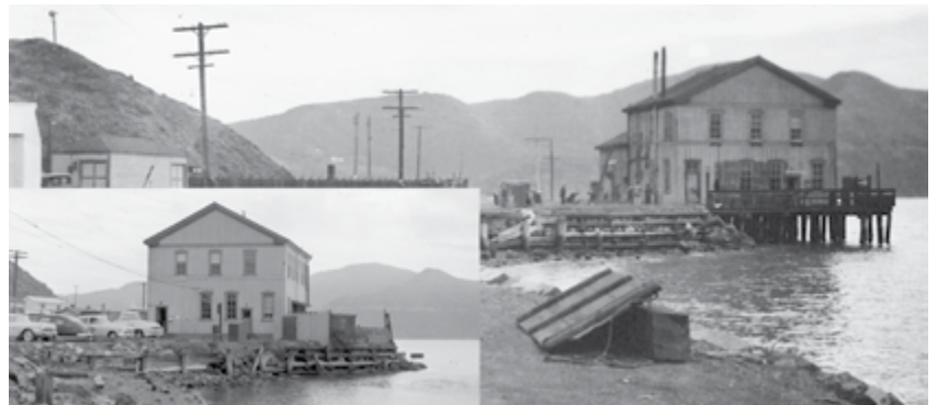
The Depot building was moved off its dock pilings onto the shore in the early 1940s. These photos show prior to the move and afterwards in 1957.
