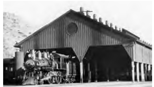
Fires caused by engine sparks, machines and human carelessness were a constant fear at the rail yards during hot, dry summers. So most of the large buildings like the passenger shed, photographed here in 1909, had rows of water barrels perched along the roof line with ropes attached on both sides that could be pulled to dump the water.
